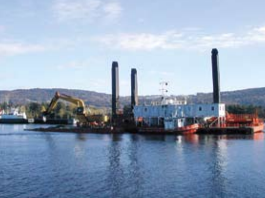
Borerigg for undervannsarbeid.
